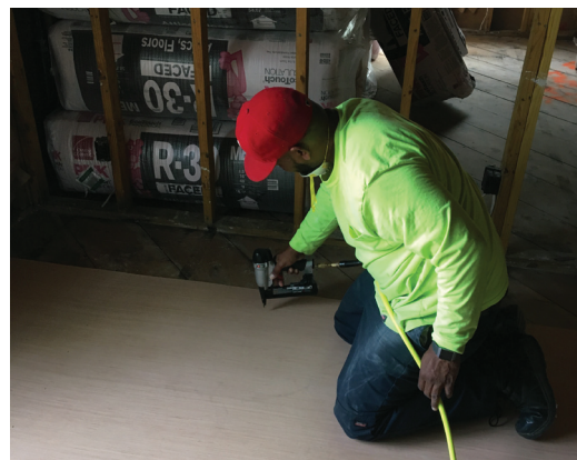
Larry Waddell works to secure flooring in the house.
