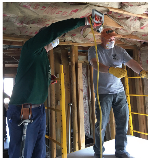
Ken Plummer and Richard Everett install insulation in the ceiling of the home.
