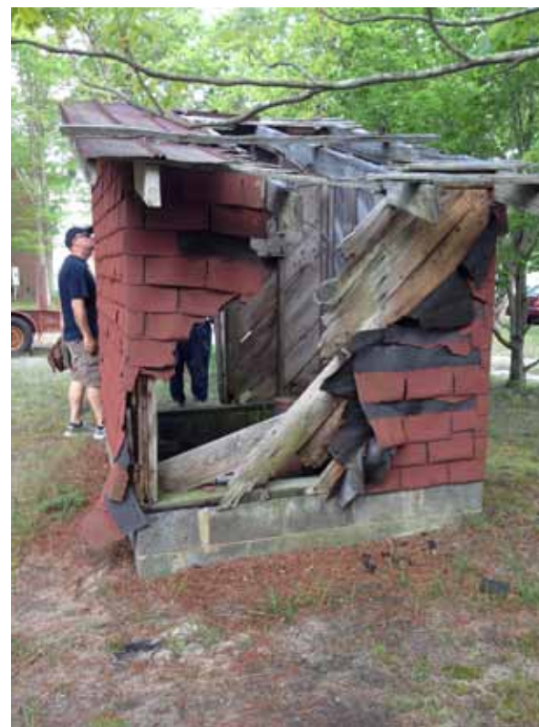
Back of pump house before restoration, roof and back wall extensively damaged, many support beams water damaged.
